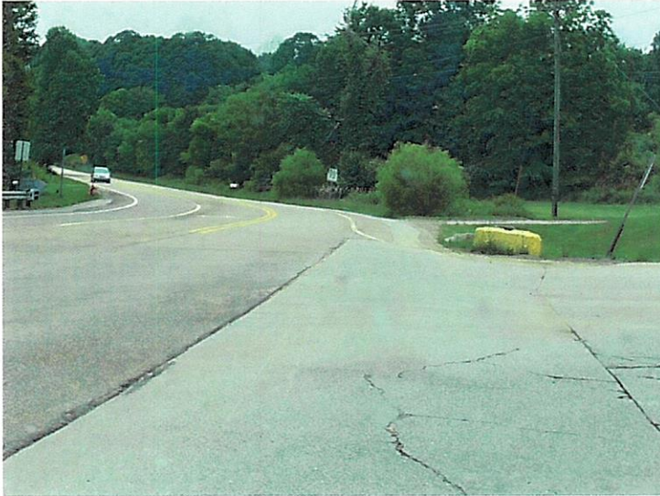
view of HWY 72 gate entrance
