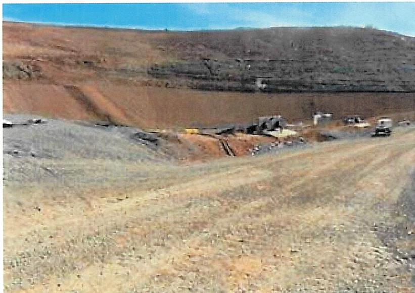
View of new cell (not in active use but approved by DSWM). Site still utilizing upper existing corner. Plan to divert soft msw loads into cell discussed and need for 2 working faces for few weeks acceptable-new expanded dump pad corner in view to left. Some wind blown litter visible-personnel found this time recovering. Pumps at risers set for active use. Continue effort.
