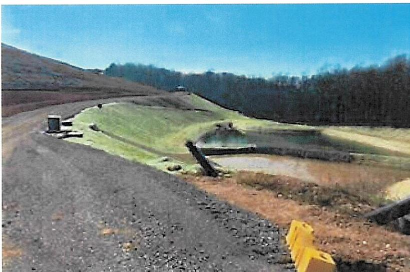
view of new adjusted pond with grass emerging on banks as stabilized.
