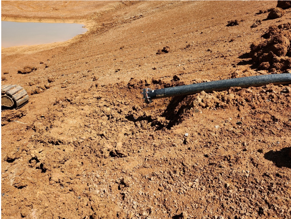
SITE PHOTO 1 – EXPOSED LEACHATE DISCHARGE PIPE PRIOR TO UNCAPPING
