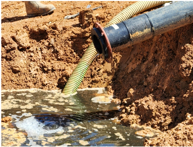
SITE PHOTO 3 – TYPICAL FLOW FROM LEACHATE PIPE AFTER UNCAPPING AND RELEASING INITIAL HEAD
