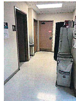
Prep and Repaint Interior
