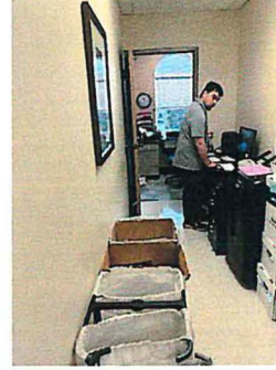
Prep and Repaint Interior
