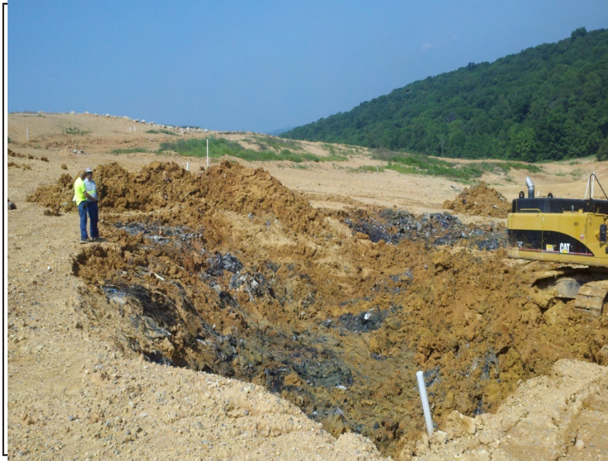
Photograph 9: View looking South of formerly depressed area after soil cover removed to expose waste and sludge.
