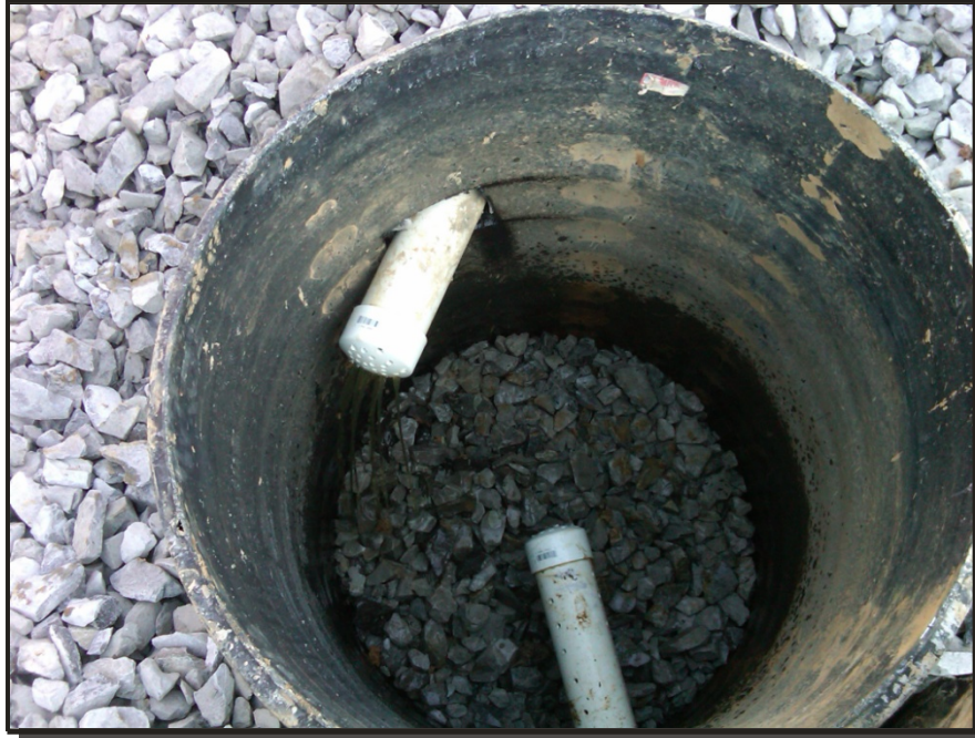
Photograph 1: Condition of base of vertical riser pipe in the LCS at bottom of Module G
