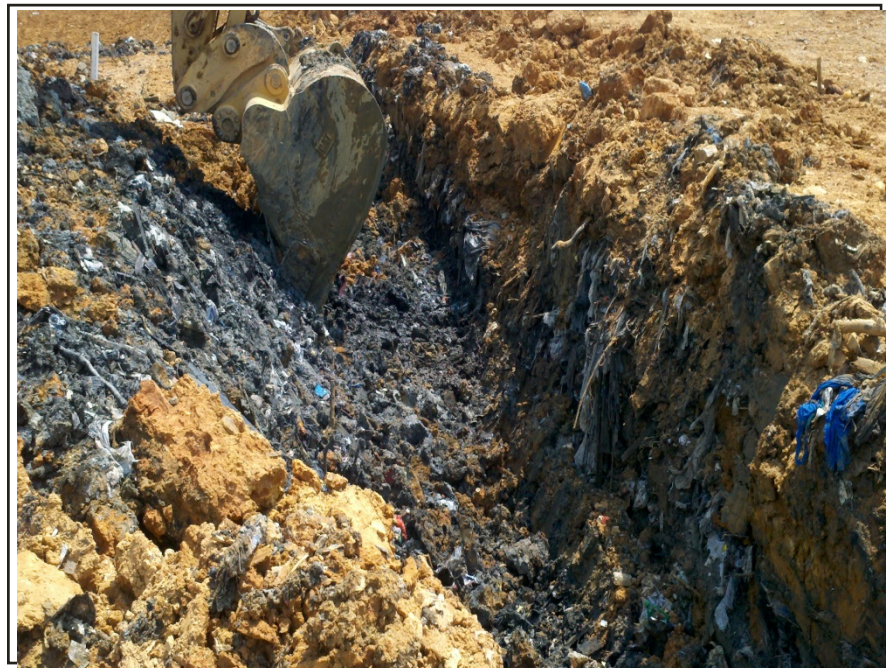
Photograph 14: Excavated trench continuing to advance southeast and approaching the scarp area. The sludge layers are reported to be approximately 8-ft deep in this area which is then underlain by relatively dry waste.
