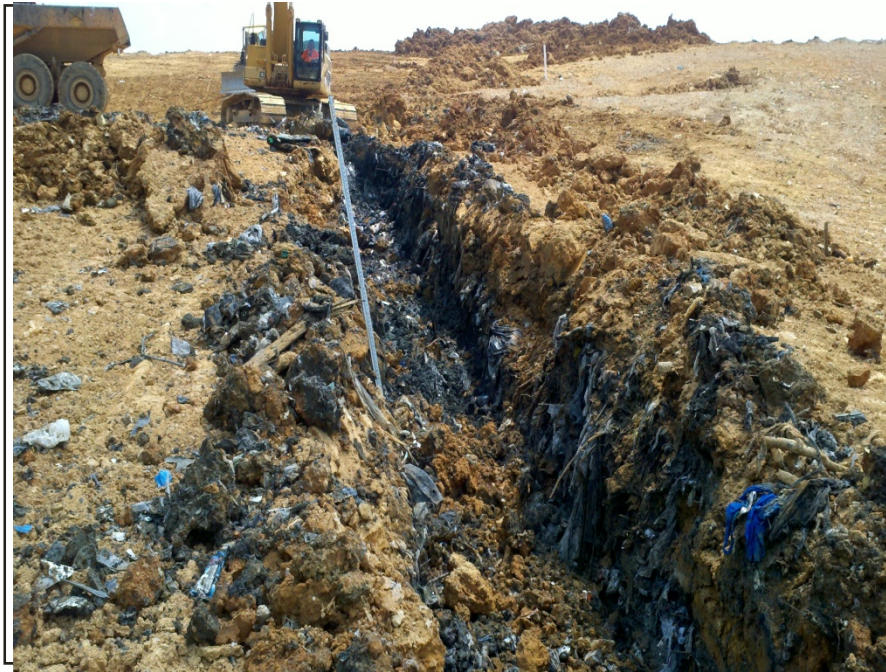
Photograph 13: Excavated trench progressing towards scarp area. Note that sludge is being encountered in this area.
