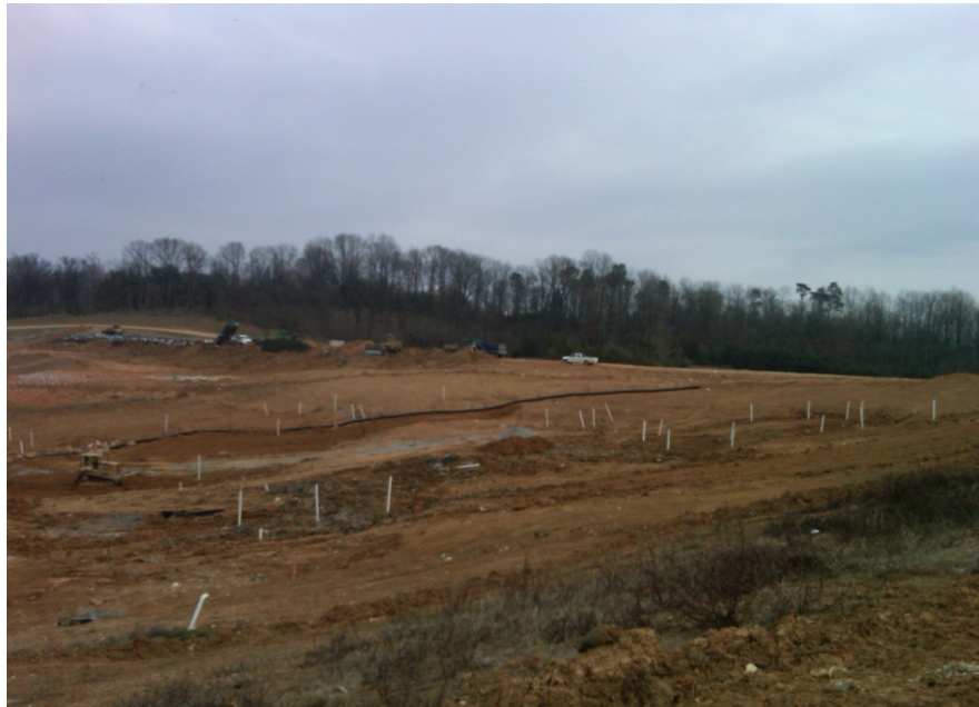
Photograph 6: Indication of the density of drains and gas vents in upper reaches of Module G.
