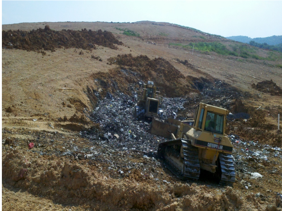
Photograph 11: View of waste being excavated. Santek reported that once sludge was removed (See Photograph 9 and 10), the underlying waste was relatively dry.
