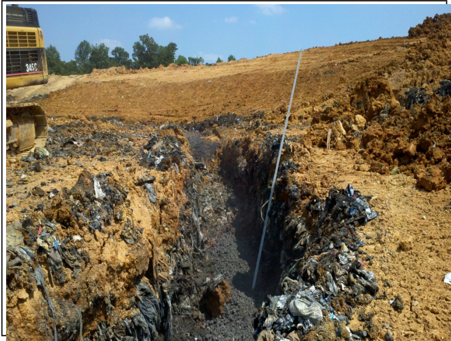
Photograph 15: Excavated trench near the edge of the former scarp area. Gravel is placed in the trench to promote drainage to bottom of cell.
