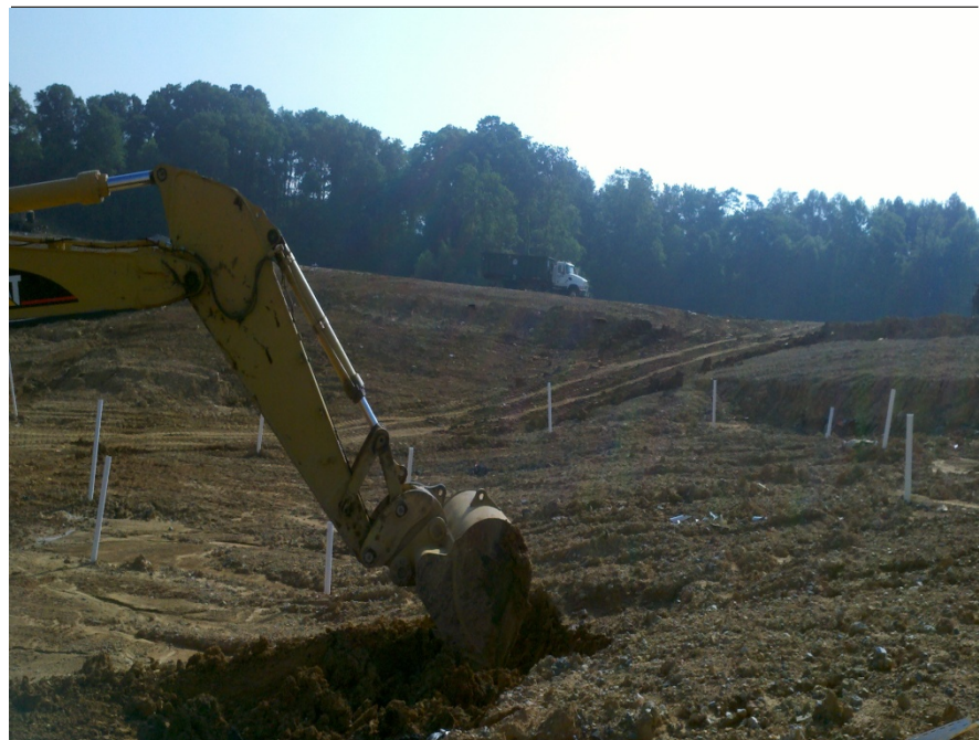
Photograph 8: Area where depression repeatedly appeared prior to commencement of excavation. Notice that gas vents and drains had been previously installed in area to be excavated.
