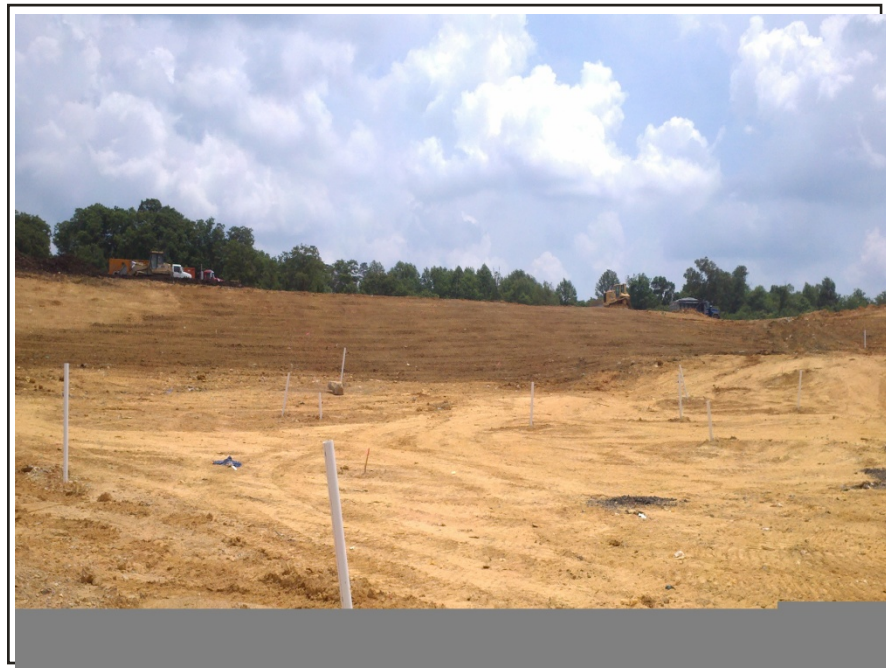
Photograph 18: View of former scarp area upon completion of excavation and regrading.
