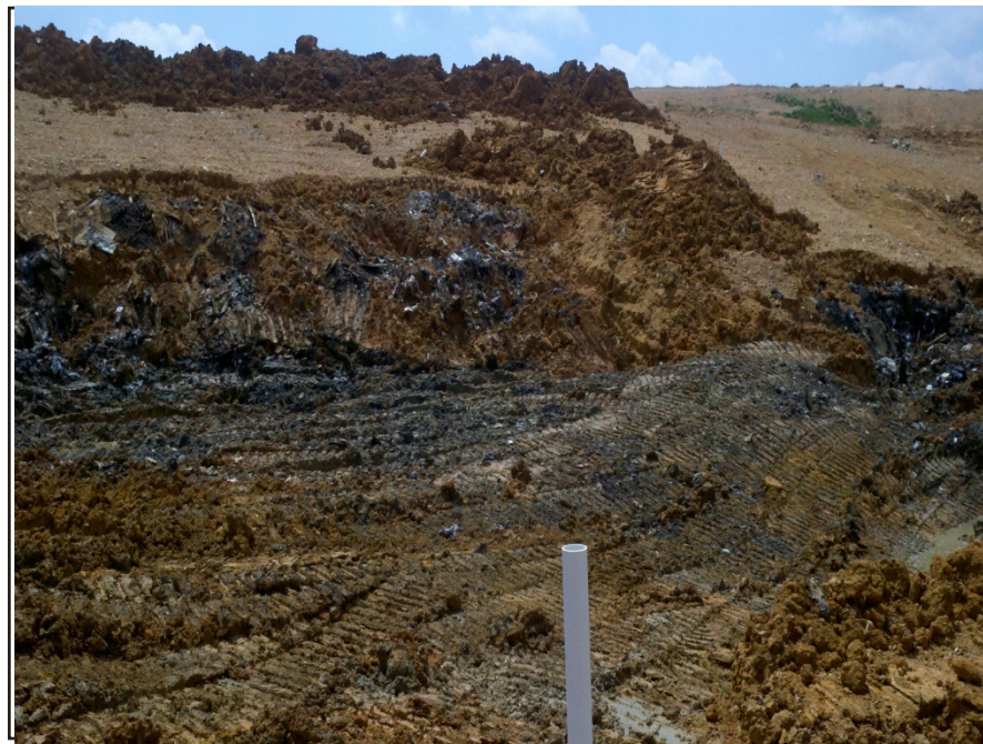
Photograph 10: View looking East of formerly depressed area after cover soil was removed to expose waste and sludge.
