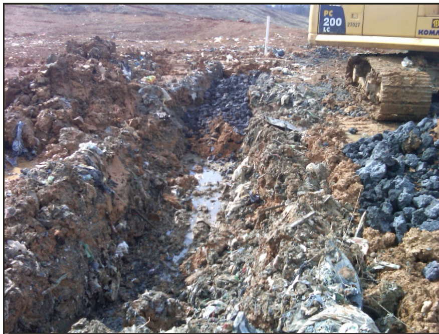
Photograph 4: Close-Up of excavated drainage trench showing liquid in bottom of trench, gravel that has been recently placed, and an installed gas vent.
