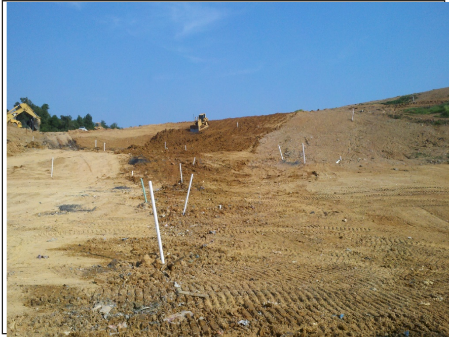
Photograph 17: View looking South to show installed drains/gas vents and placement of intermediate cover in excavation areas.
