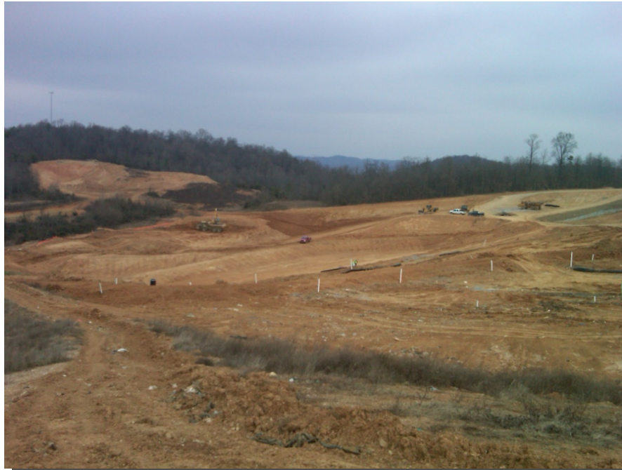
Photograph 7: Indication of drains and gas vents in lower reaches of Module G and stormwater diversion berm near base of cell.
