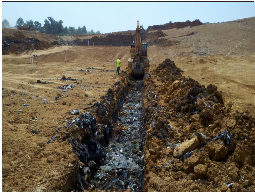
Photograph 12: Excavation of drainage trench from existing drainage trench towards the excavated (and now covered) area where sludge pockets were encountered.
