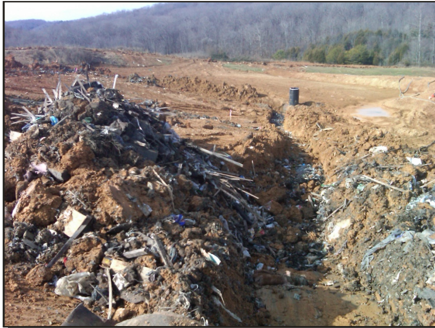
Photograph 3: Excavated Drainage Trench looking towards bottom of Module G. (Note the repaired vertical riser near bottom of cell)
