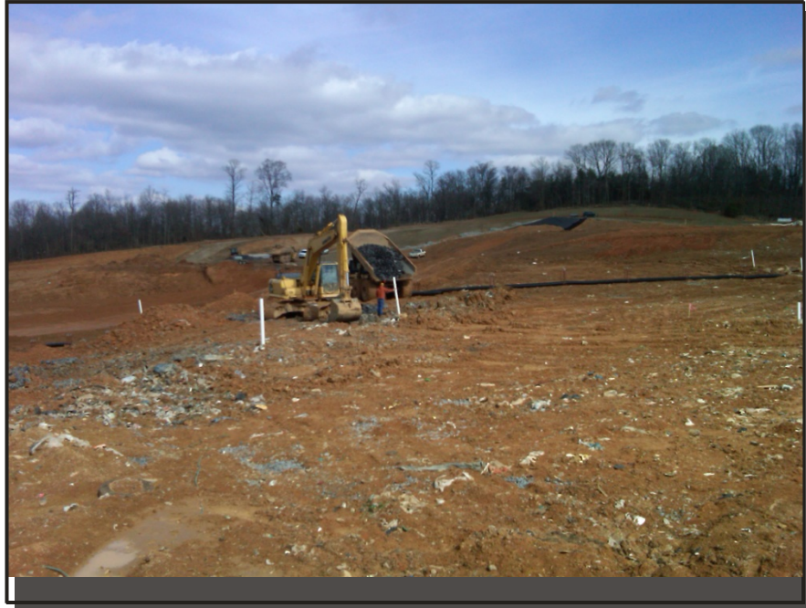
Photograph 5: Down-gradient progression of gravel placed in trench adjacent to gas vent and surface completion of trench to minimize direct percolation of surface water.
