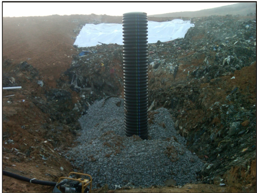
Photograph 2: New vertical riser pipe and gravel in the LCS at bottom of Module G
