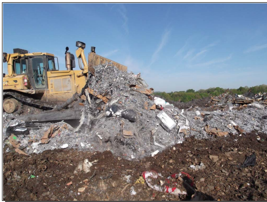
Photograph 2: Mixing MSW with K-C RFD material.
