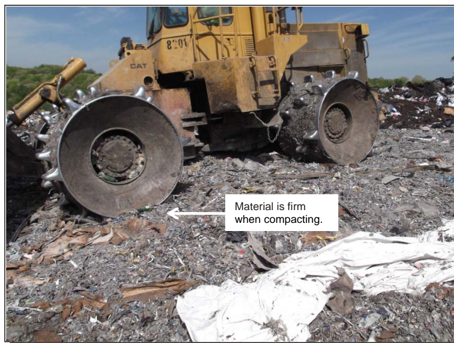
Photograph 4: Compacting 50% MSW and 50% K-C RFD material.
