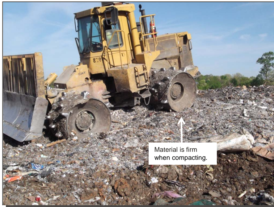
Photograph 3: Compacting 75% MSW and 25% K-C RFD material.
