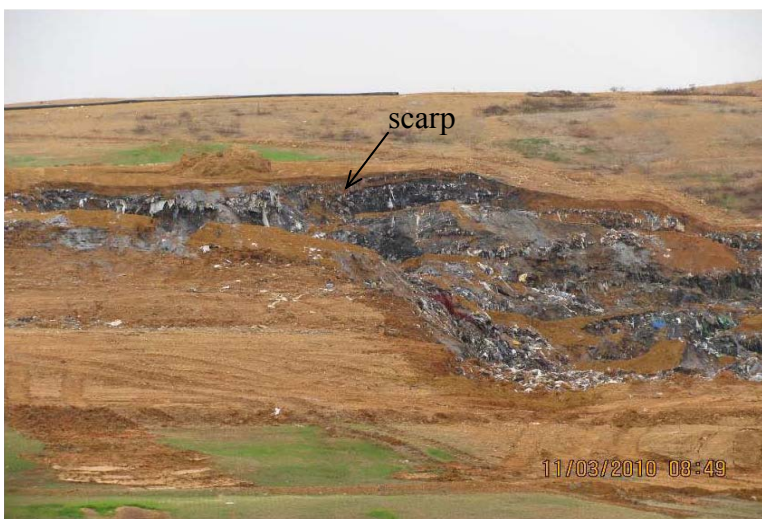
Figure 1. View of the Failure Area Near the Toe on 3 November 2010
