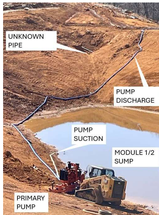
Figure 4: Leachate Disposal System (Primary Pumping System)
