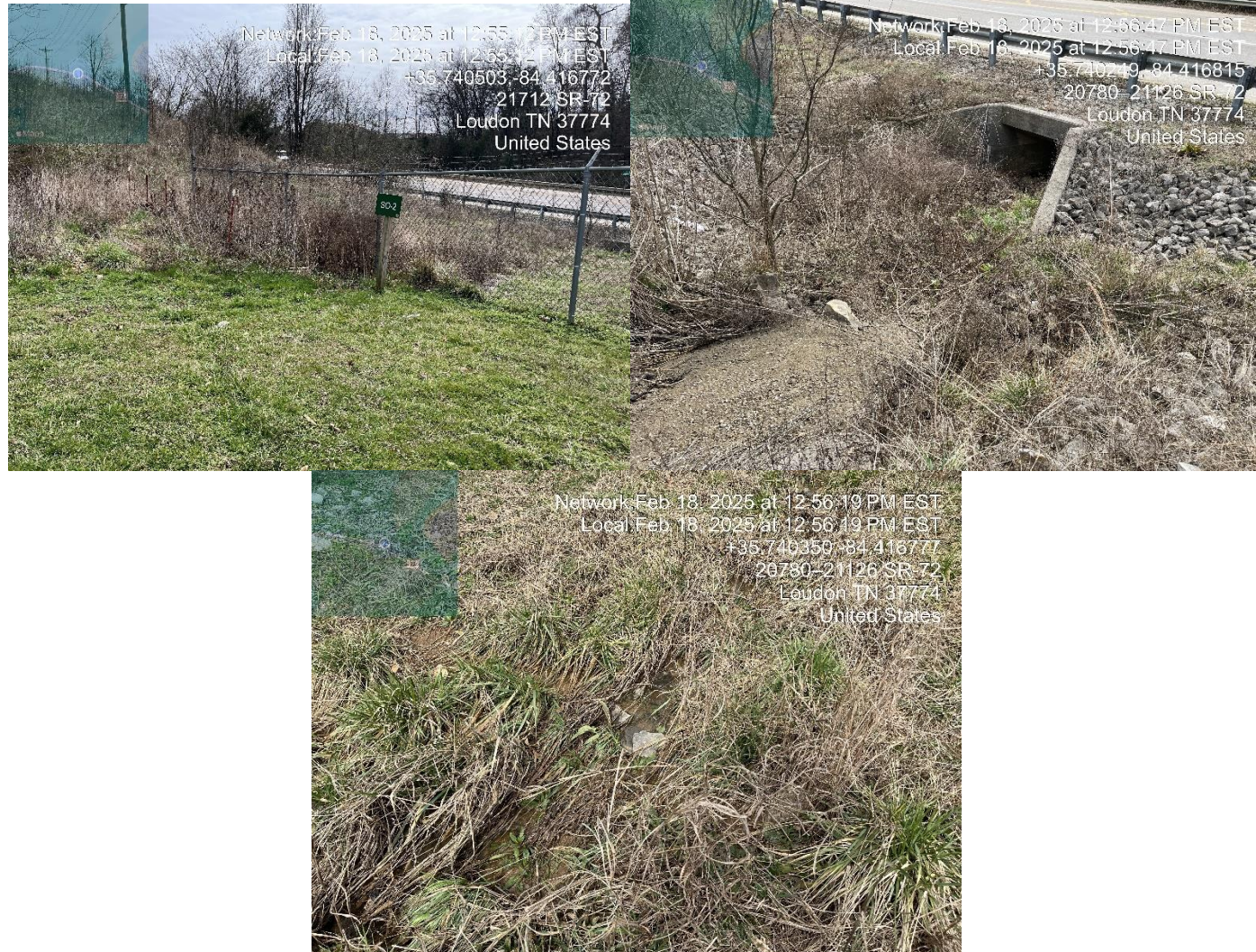
Outfall 2 (SO-2): Area is vegetated and riprapped. Discharge observed was clear.
