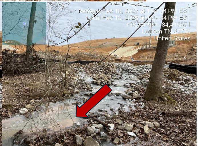
Outfall 3 (SO-3): Sediment Basin under active construction to expand-see CGP Inspection Report. Discharge treated with riprap, filter bag and silt fence. Stand pipe to be installed as soon as weather allows. Discharge appeared clear. Small sediment depositions (red arrow) observed but do not appear recent, as current discharge was clear and no sediment staining was observed on the riprap filter.
