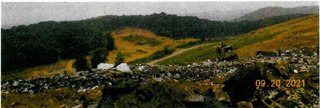
View of working face from right (upper photo) to left (lower photo), panning away from area where trucks are dumping. Due to the shape and location of the working face on the slope, it was hard to photograph from the top of the slope. The working face was cut into the slope below, which made it well-contained and a manageable size.
