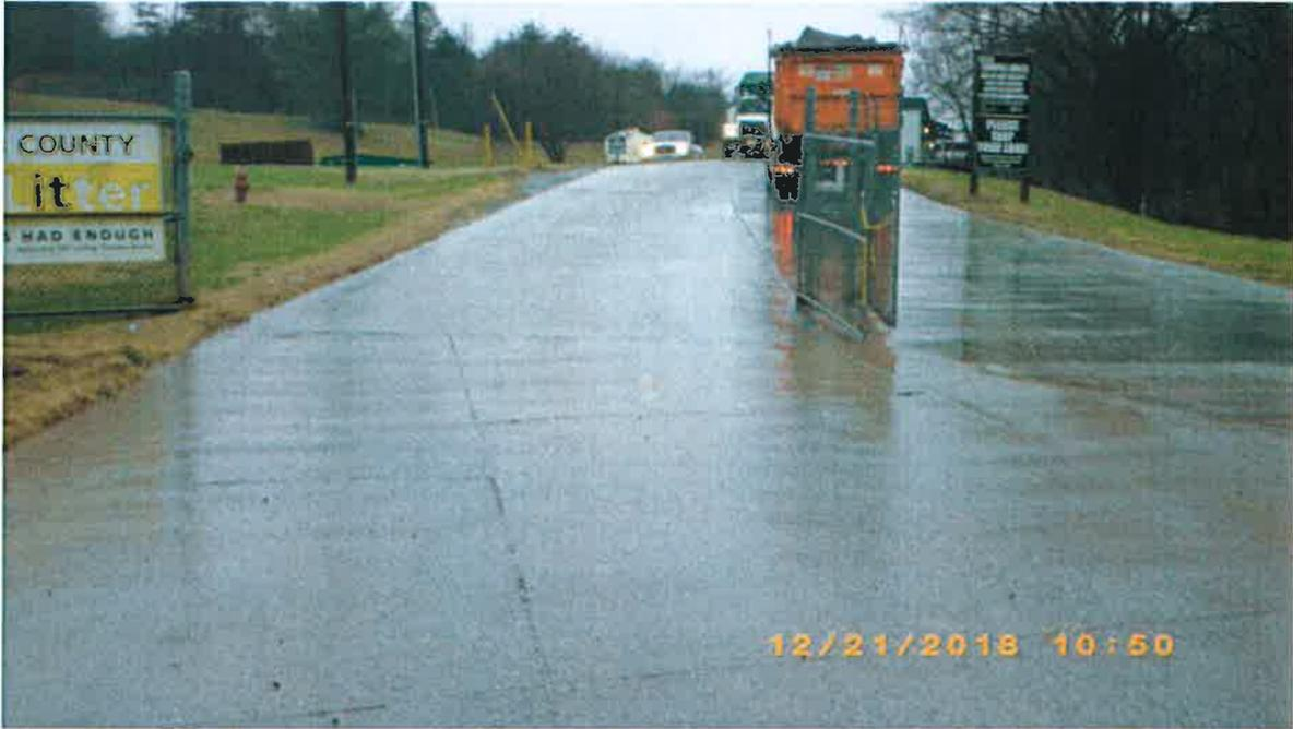
Landfill driveway. Sheet flow runoff observed. No siltation, mud or rock observed.
