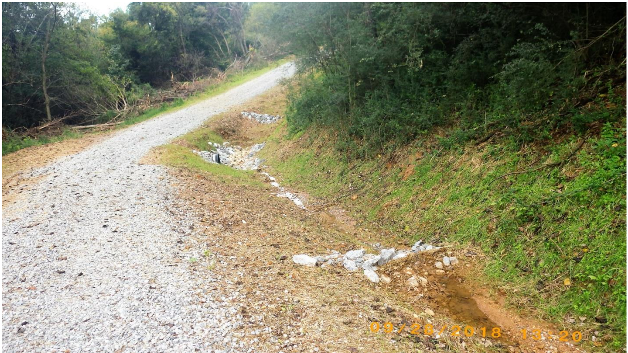
Check dam after hard rains of 9/25 & 9/26/2018
