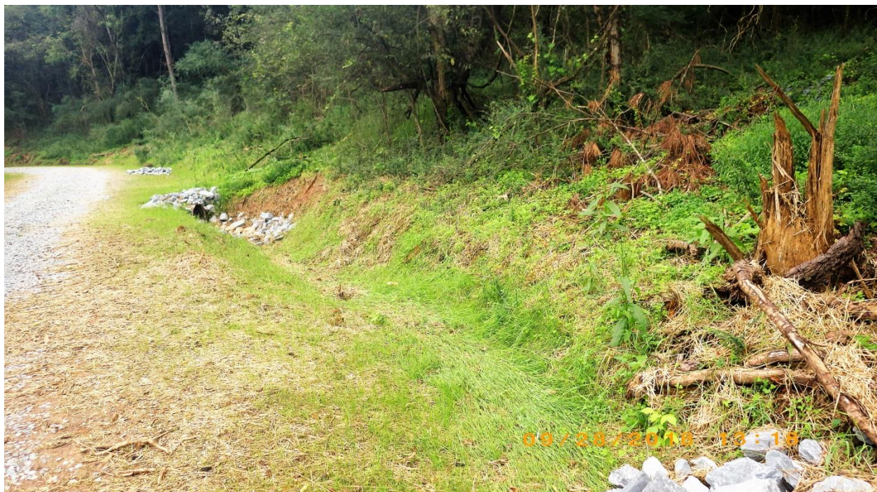
Drainage way showing grass laid down from hard rains of 9/25 & 9/26/2018.
