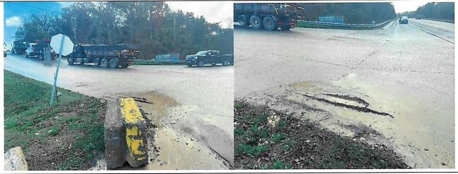
During the investigation, sweepers were seen actively clearing mud off the roadways. Sediment was also observed accumulating around the entrance/exit and staining was observed across Highway 72. This issue is noted to be ongoing. A preventative solution is needed to remove any material on tires prior to leaving the site. Consistent tracking of mud can potentially cause a condition of pollution in Waters of the State, a violation of the *Water Quality Control Act of 1977*.
