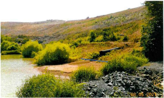
Photo of this area from August's inspection, for comparison. Sediment beyond blue line/true perimeter of pond needs to be completely excavated and removed to a location where it will not be washed back into the pond.
