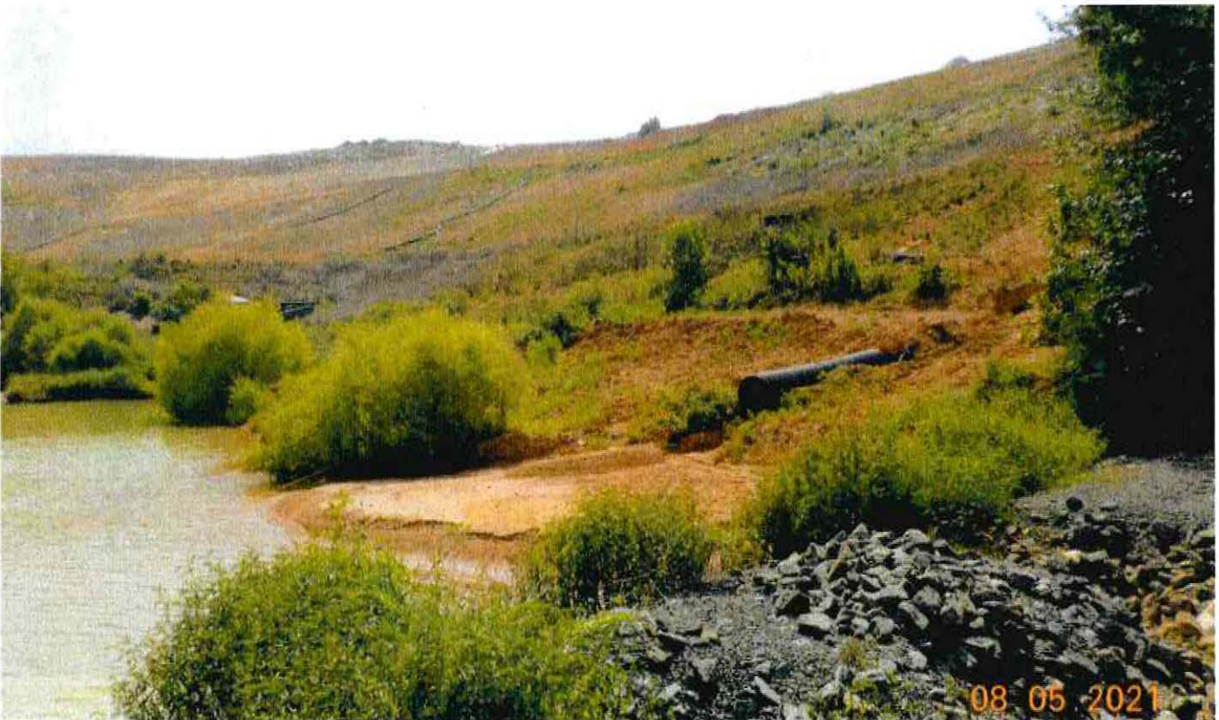
Lots of sediment accumulation in some areas of the pond, such as this spot where water enters the pond through a pipe. Sediment here has accumulated above the water level in the pond. Pond clean-out is in progress. An approximate timeline of the end of August for completion of the cleaning was discussed during the July inspection.
