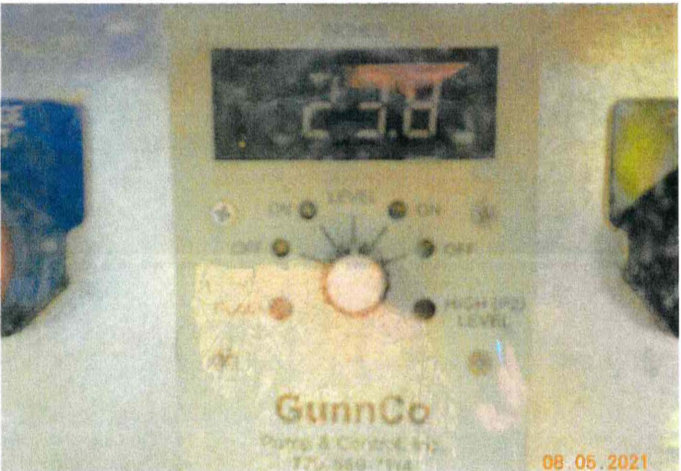
Leachate head reading at sump was 23.8", which is in compliance.
