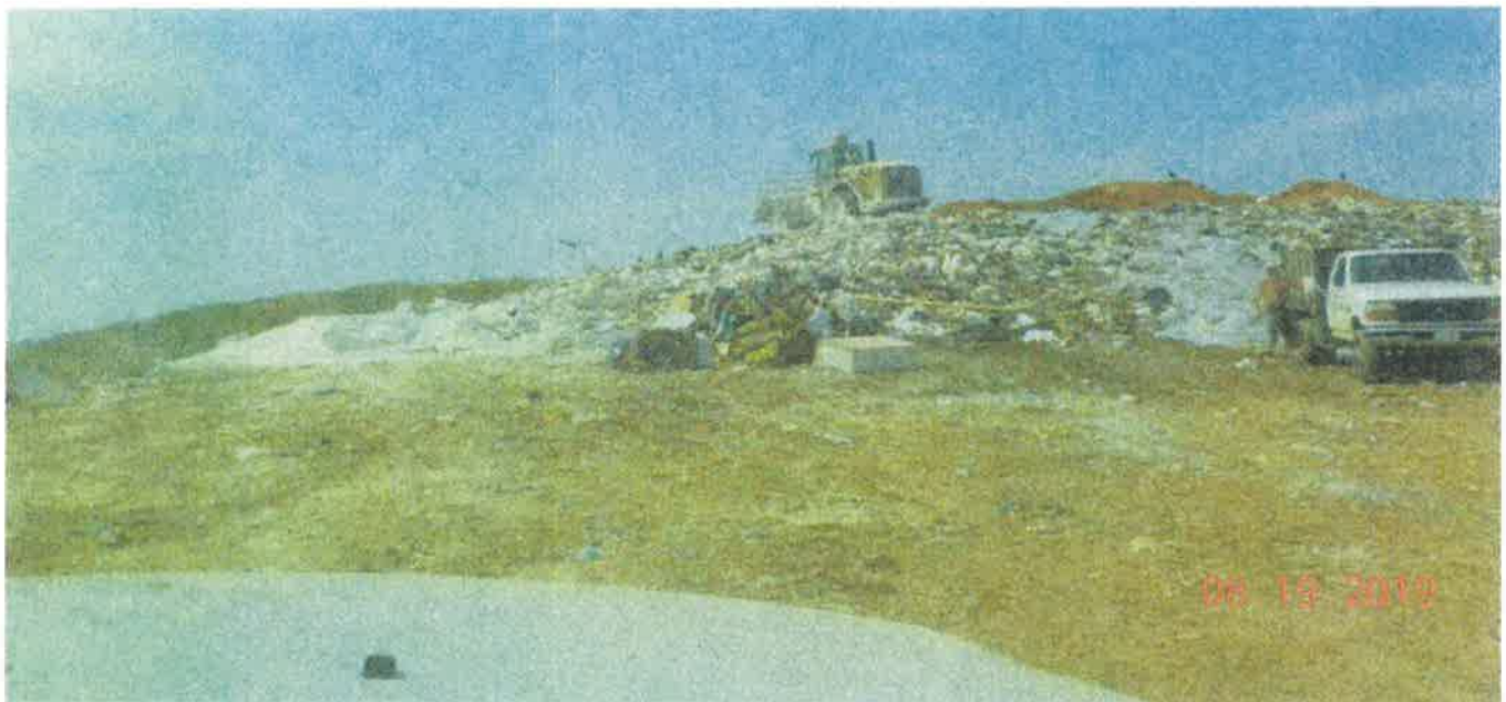
Left side of working face. White material is "clay" from make-up product.
