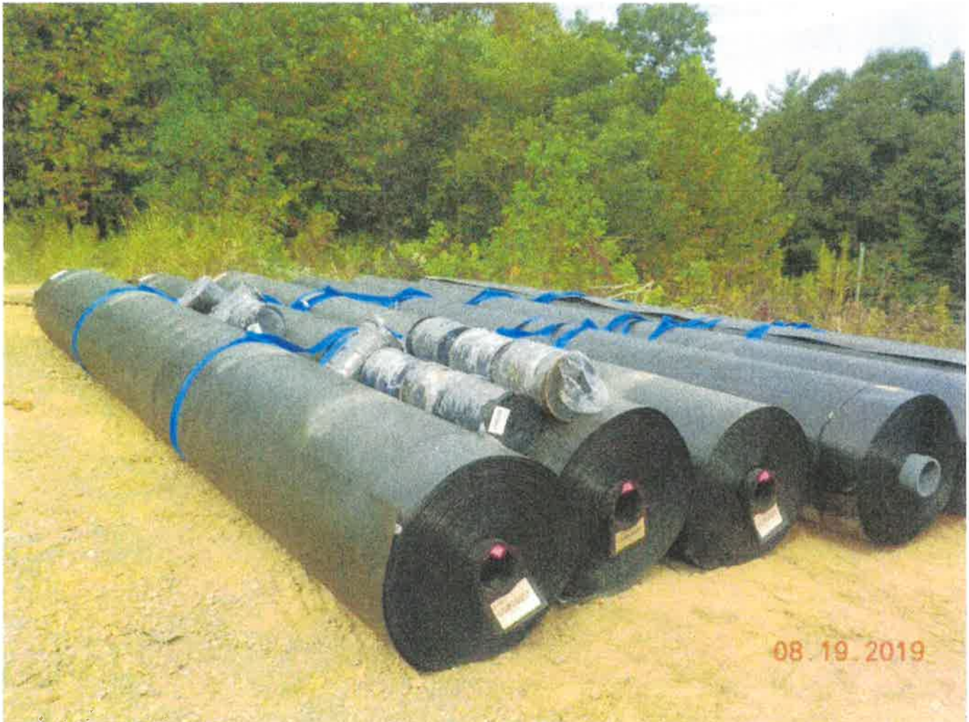
Rolls of plastic liner for new cell.
