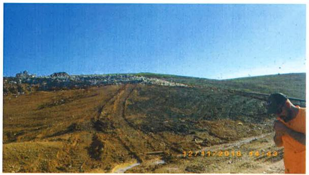
Working face looking south from toe. Soil cover stockpile behind waste placement.
