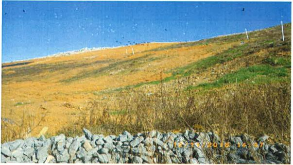
North slope leachate seep repairs functioning well.
