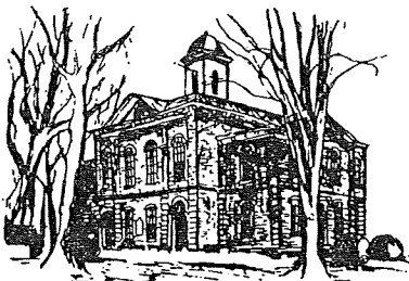
LOUDON COUNTY COURTHOUSE LOUDON, TENNESSEE ERECTED 1872
