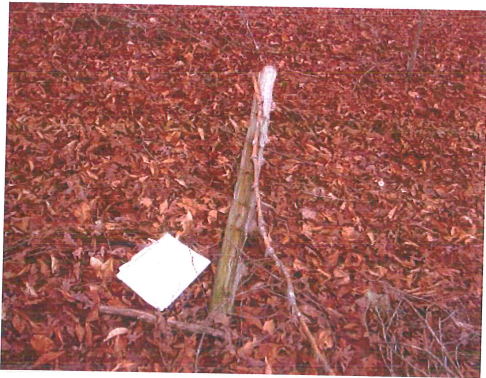
Photo No. 14: Atchley Property – Downed fence line along Atchley-Ryan property line vicinity of southeast corner.
